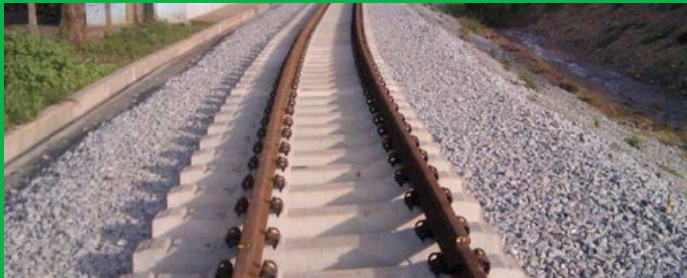
Newly completed Sekondi-Takoradi via Kojokrom Railway Line
