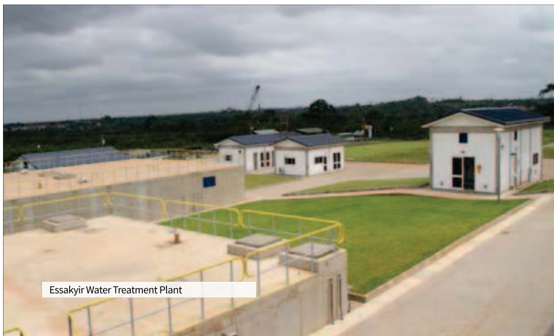
Five Towns Water Supply project
